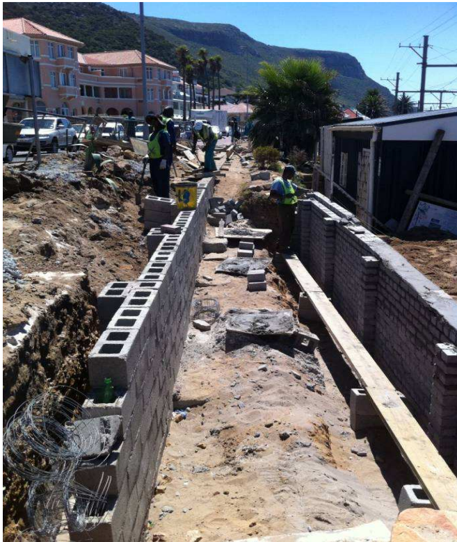
PLUMBING AND ACCESS RAMP AT HAVEN NIGHT SHELTER
